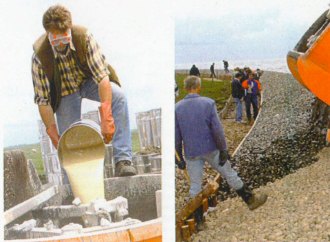
Gravel are coated with Elastocoast® in a standard mixer
